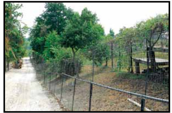
This photo shows the current perimeter fence. As you can see, it needs to be rebuilt to keep the wild animals out. Please help.
